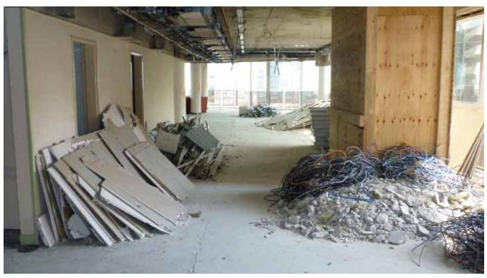
Gypsum sticks to other construction materials in demolition waste, making it difficult to valorise the material
