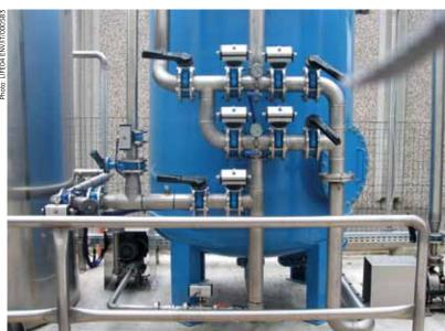
Treated wastewater was re-used effectively in a range of production processes from fabric softening to some washing processes and overall the project demonstrated that fresh water consumption could be reduced by 40% on an industrial scale, with a five year return on investment.
